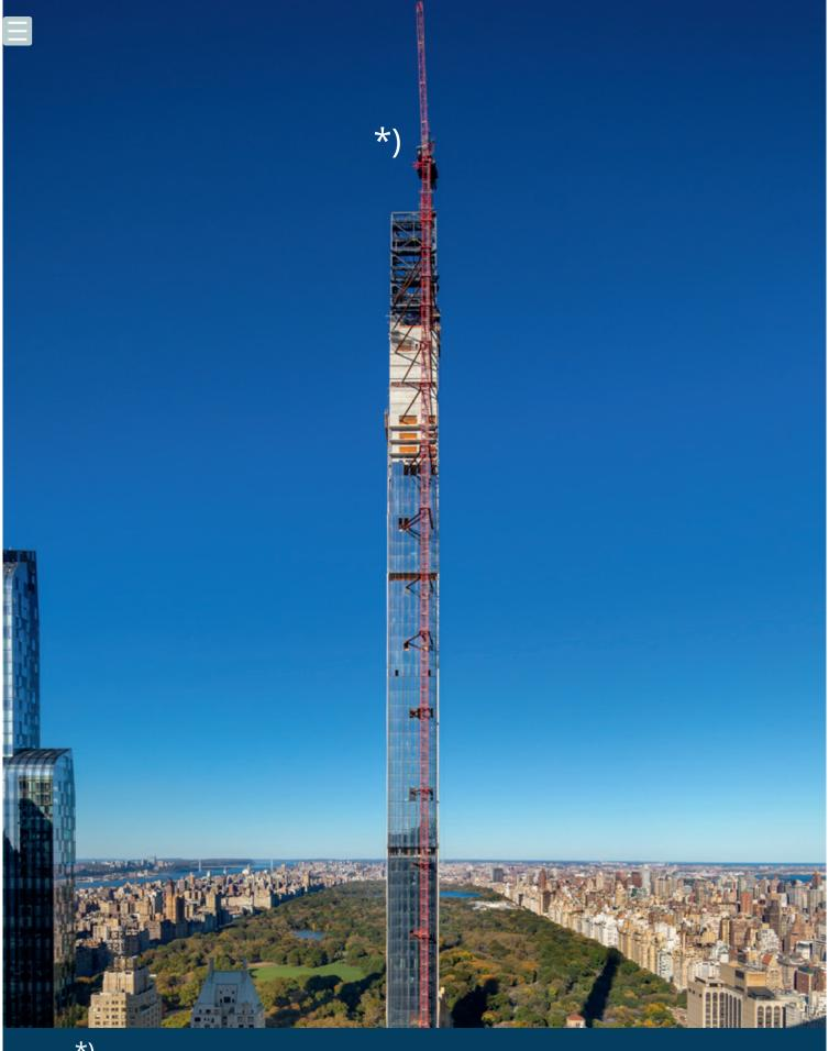
New dimensions. In New York, the world's narrowest skyscraper is being built to a height of 435 meters. The Steinway Tower reached its full height in 2020 and is scheduled to be ready for occupancy in 2021. With a height-to-width ratio of 1:24 (the usual is 1:7), the tower, which will house around 60 luxury apartments, not only plays with dimensions, but also places the highest demands on construction.
